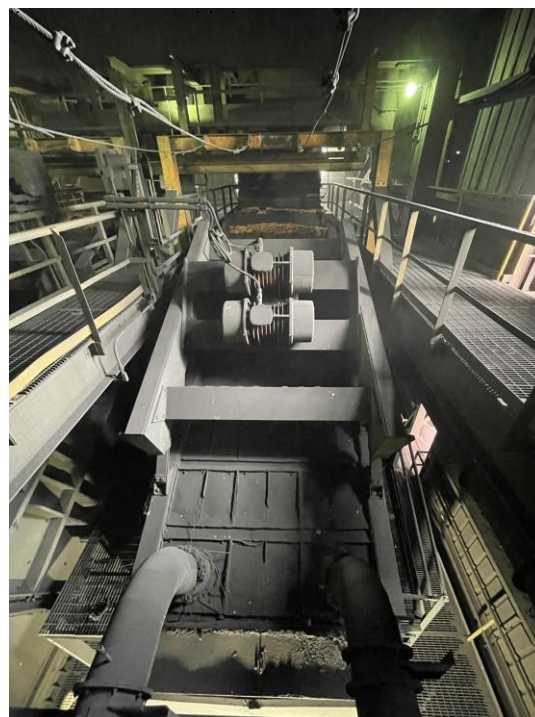
FIGURE 7: SCREENING DRI PRIOR TO SHIPMENT
