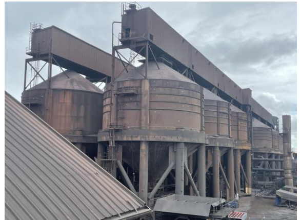
Figure 4: DRI storage silos Image courtesy of Nulron
