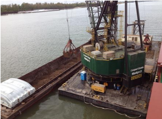
FIGURE 23: BARGE "SOFT LOADING"
